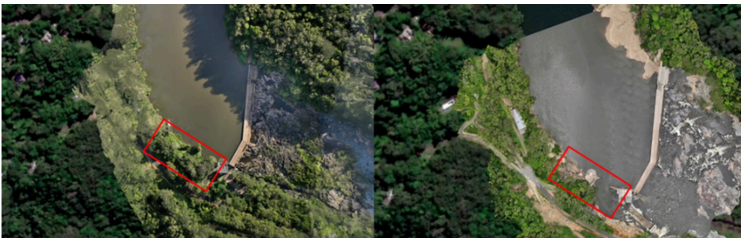
Figure 2. Before and after 2023 floods, note the bank and access to the intake tower that was washed away (inside red box) and sand deposited on the northern bank.
