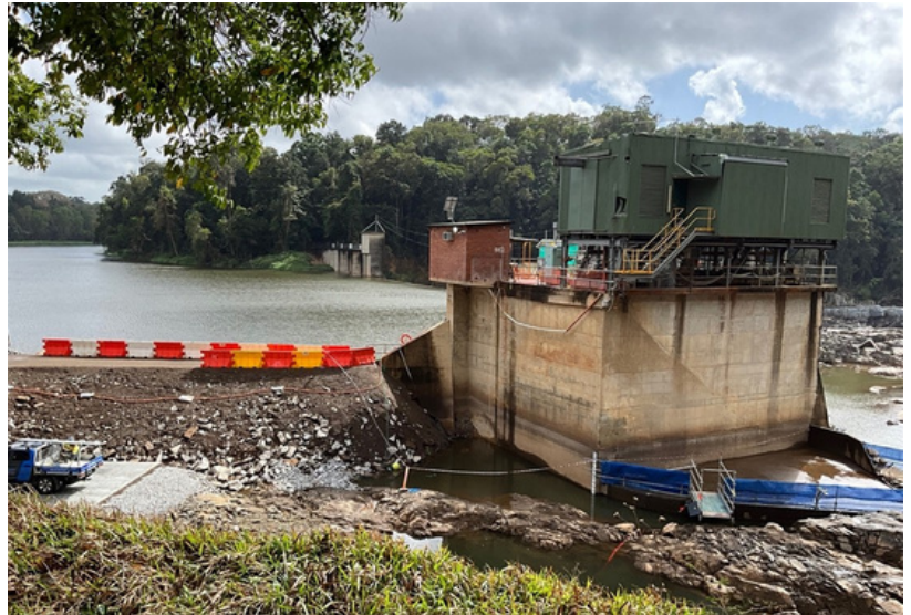
Figure 3. The Barron Gorge Hydro Station intake tower and temporary access wall.
